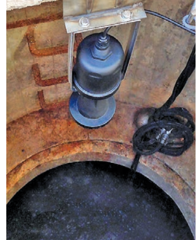
The LR30 pulse radar sensor is the reliable level measurement solution for municipal and industrial pump lift stations.
